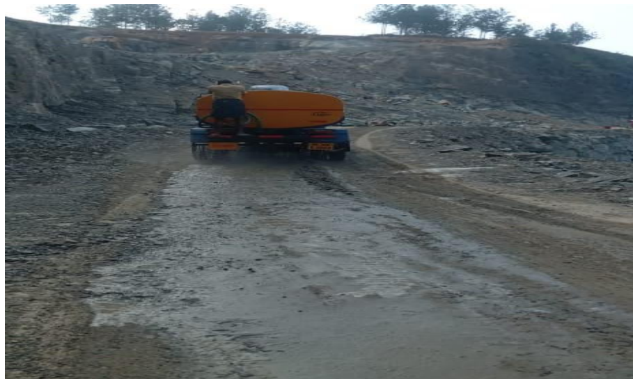
Figure:5 Photographs showing water spraying on quarry road for dust suppression.
