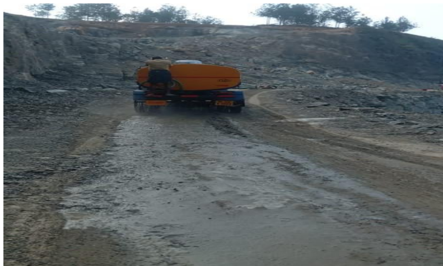
Figure:4 Photographs showing water spraying on quarry road for dust suppression.
